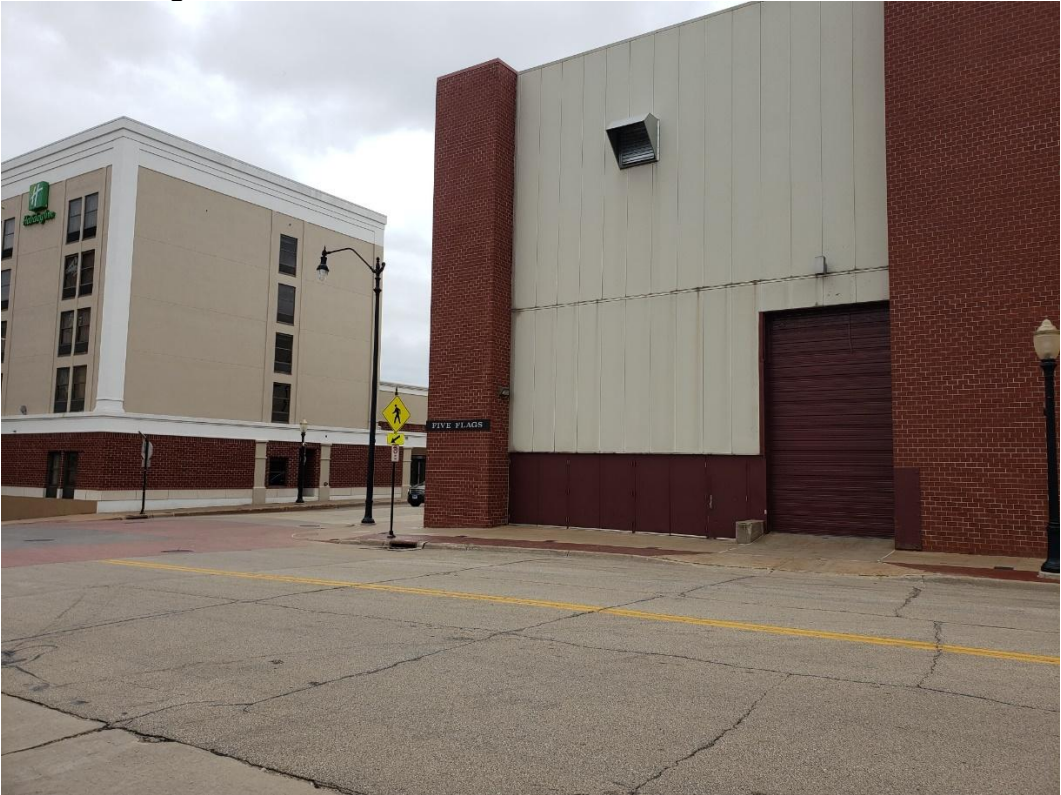
Fifth Street Loading Dock:
