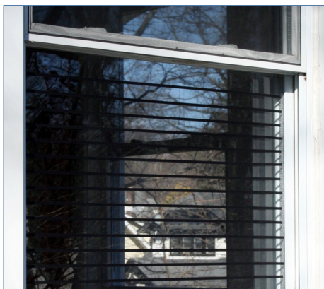
Horizontal stripes spaced two inches apart are an effective way to keep birds from hitting your windows. Photo: Christine Sheppard, ABC
