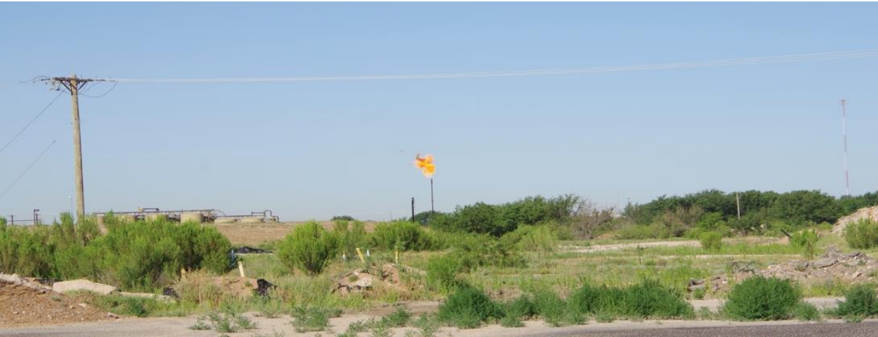
1. Adjacent tank & well
