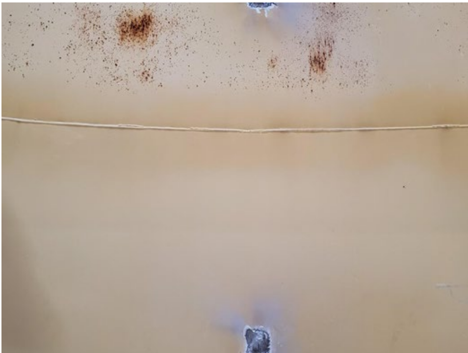
5. Interior shell angle brackets removed and ground.
