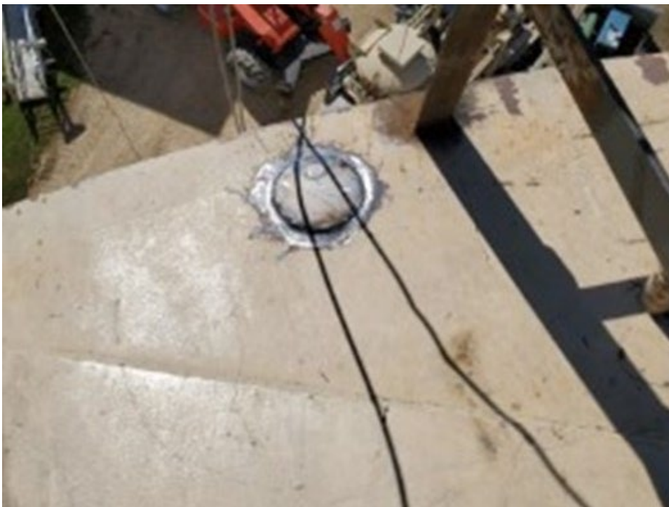
8. Roof patch plate installed.
