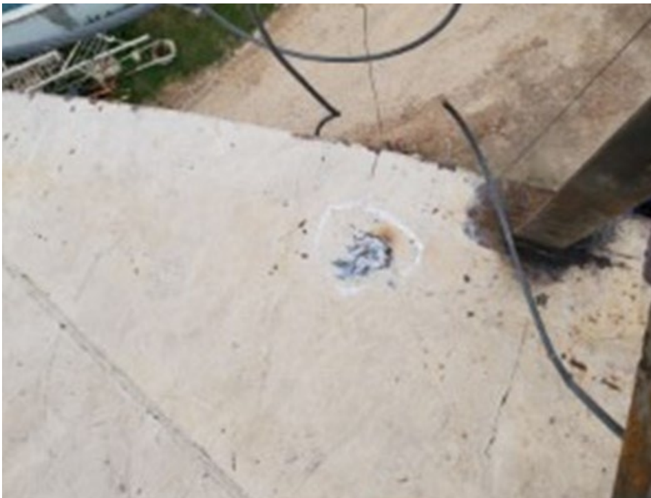
16. Exterior roof hole welded.
