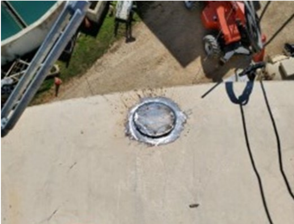
7. Roof patch plate installed.
