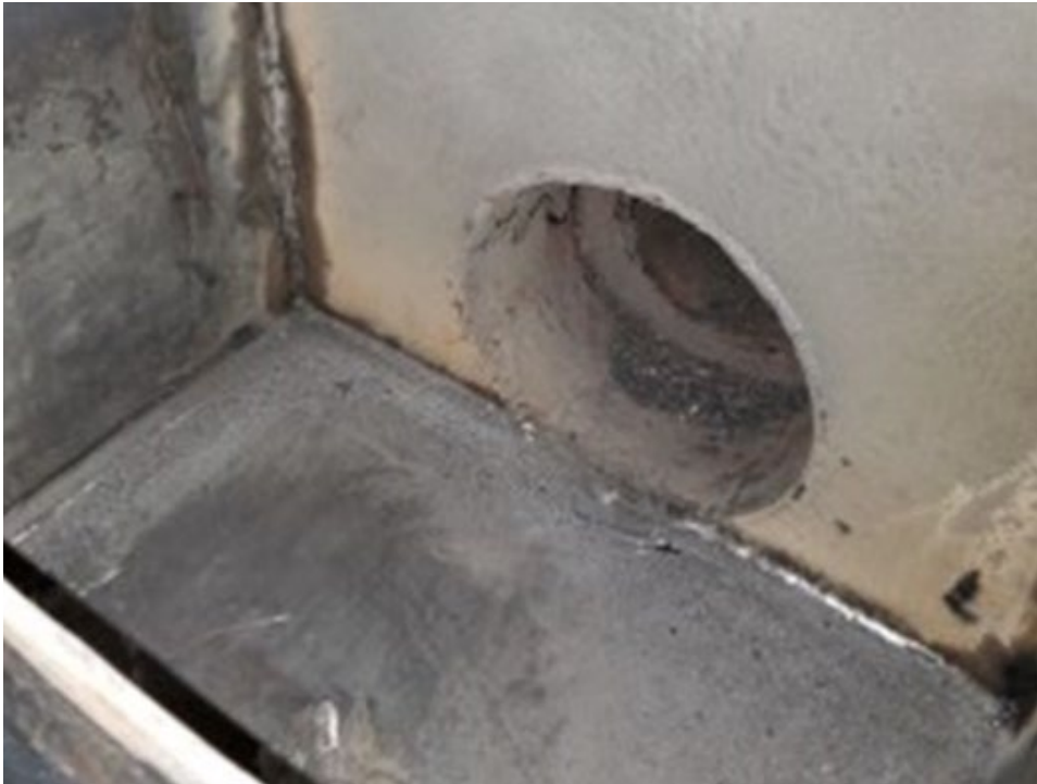
15. Interior weir box installed.
