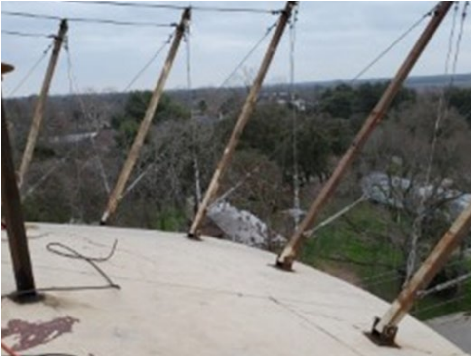
13. Exterior roof outriggers installed.
