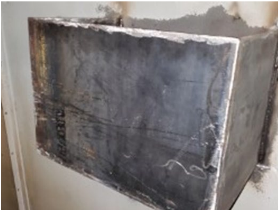
14. Interior weir box installed.
