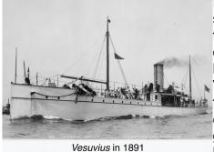
Fort Sumter. The United States Navy allowed two ships to be viewed in the harbor during the week and they were the USS Dolphin, PG-24, a gunboat and dispatch vessel and the USS Vesuvius. Both vessels had white hulls and a single stack midship. The Vesuvius was classed as a dynamite gun cruiser that fired a dynamite charge from one of three forward fixed cast iron muzzles using compressed air. These air guns were normally fired with a pressure of seven hundred fifty pounds per square inch.
