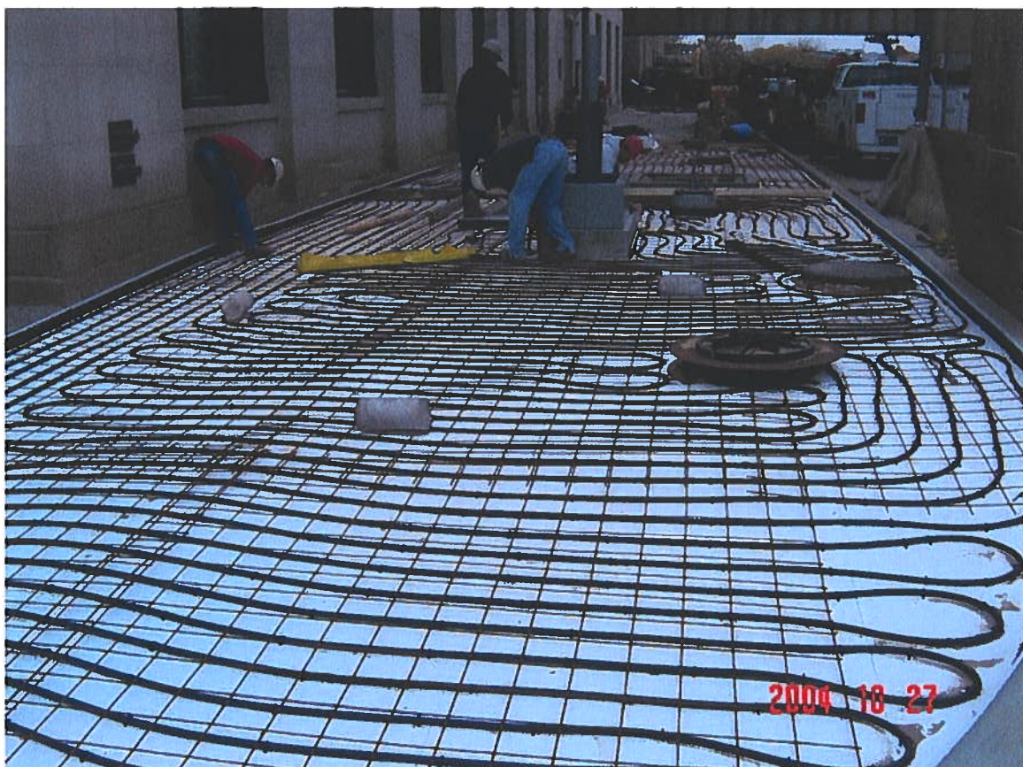
South side of Lyon Street snow melt installation.
