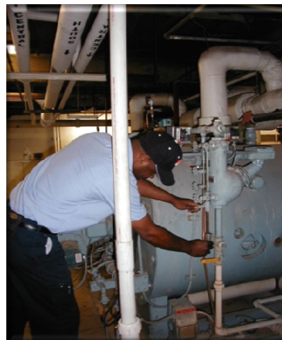
Lead Maintenance Technician, Kenny Wright, adjusts settings on the large boiler located in the basement of the Lea County Courthouse.
