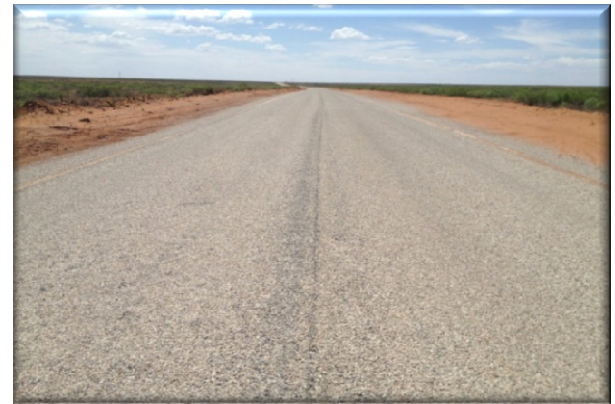
Above : County road before chip seal. Below: County road after chip seal.
