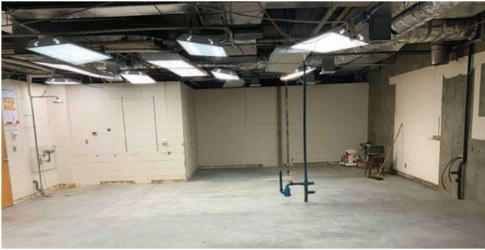
Lab space ready for renovation
