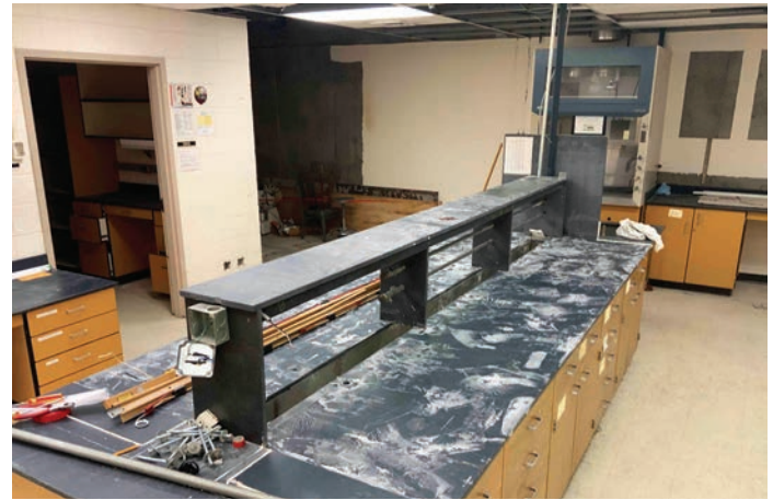
Preparing for demolition
