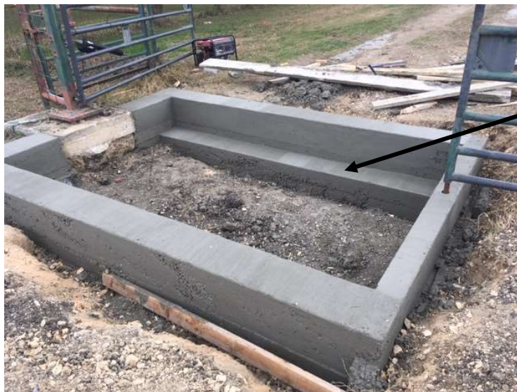
Figure 3 – Concrete Foundation including Footing
