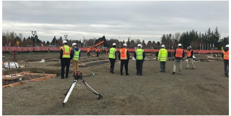
The Swinerton team leads Event Center project leadership on the first site walk.
