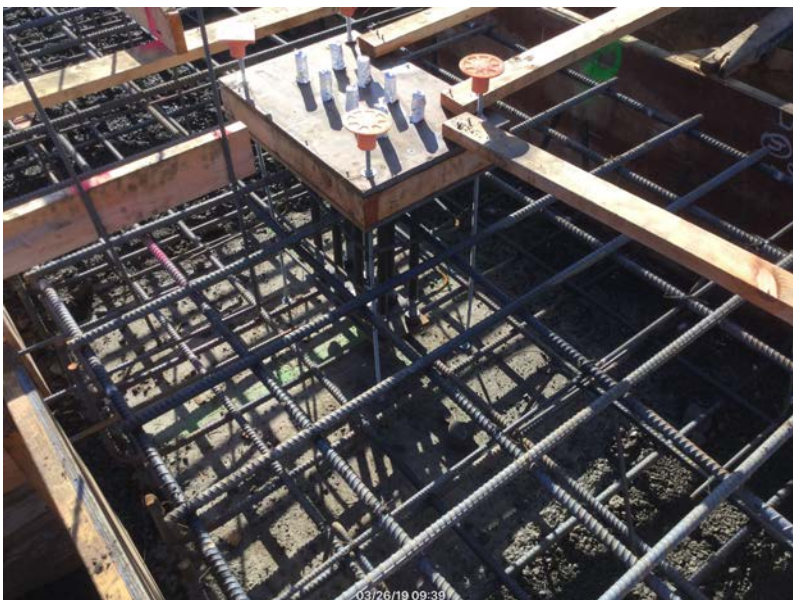
-A close-up of rebar in place, before concrete pour.
