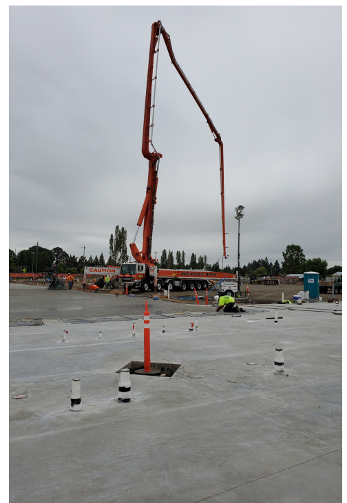
Taking advantage of a dry day to pour concrete-
