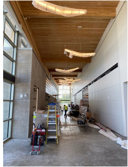
Pictured above and left - Rigorous work proceeds at the Wingspan
