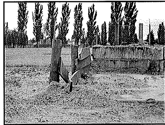
Bunker walls fractured and to be replaced.
