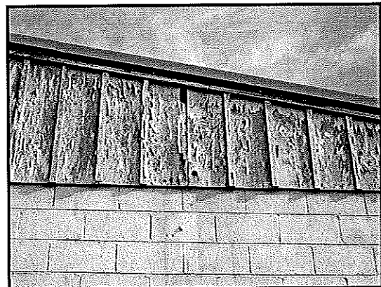
Water penetrates through cracks in wood.
