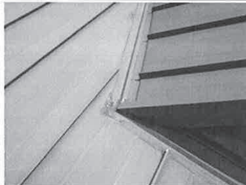
Sealant dependant cricket-to-roof connection at entrance roof.
