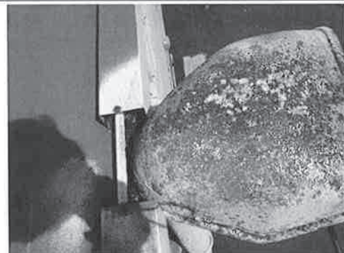
Open rake flashing where spotlight has been installed, exposing substrate to weather.
