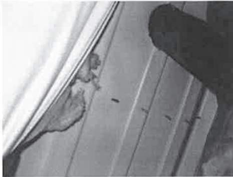
Corroded fasteners as seen from below the roof panel
