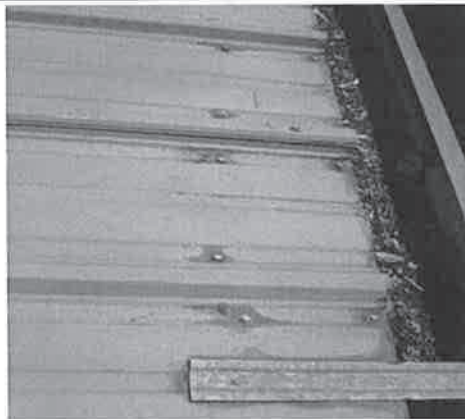
Gutter straps fastened through the roof panel. Note also excessive organic debris within gutter.
