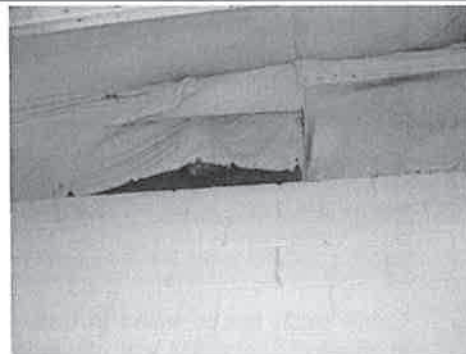
Detaching vapor retarder reveals moldy and water stained insulation at roof to wall junction.
