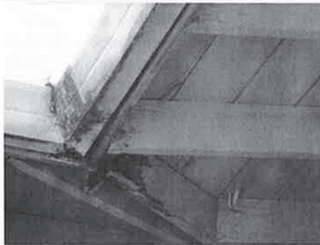
Leak at gutter seam – note stained, deformed metal and rotten wood adjacent.
