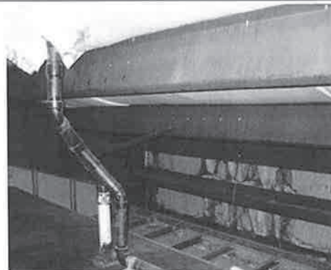
Stained and damaged wall sheathing as seen from attic space – south wall.
