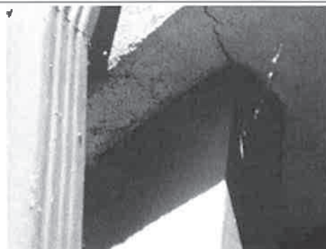
Patch/repair holes and cracks in finish system where possible.
