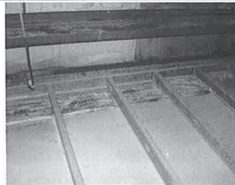
South wall – note water staining on wall and floor as well as corroded steel framing.
