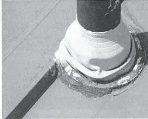
Vent pipe penetration and pipe boot flashing installed over panel seam. Flashing boot is adhered with sealant and lacks clamping and sealant at top edge.
