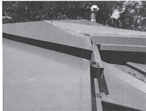
Raised ridge flashing due to detaching fasteners – south ridge juncture.
