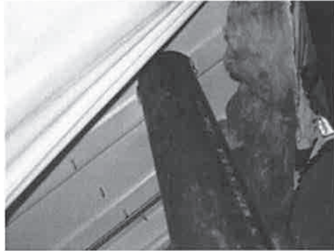
Water stained batt insulation at vent pipe penetration.
