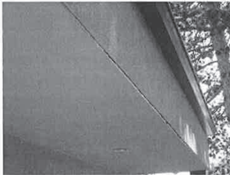
Exterior view of south wall overhang and soffit. Note soffit panel is warped and detaching from vertical wall.
