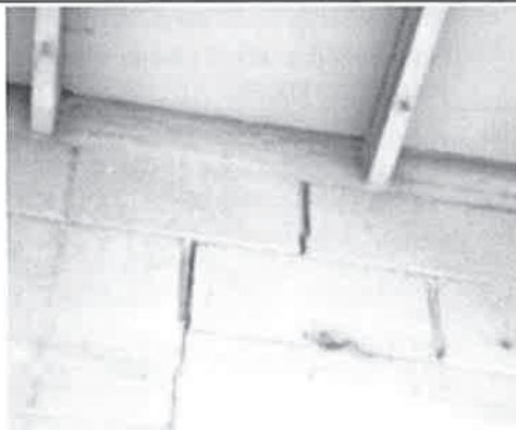
Cracks in the unreinforced concrete masonry unit wall exist at both interior and exterior of the building.
